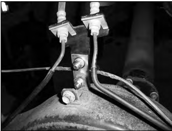
FIGURE 65A - LOOKING FROM BACK
